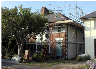
The house before the insulation was installed
